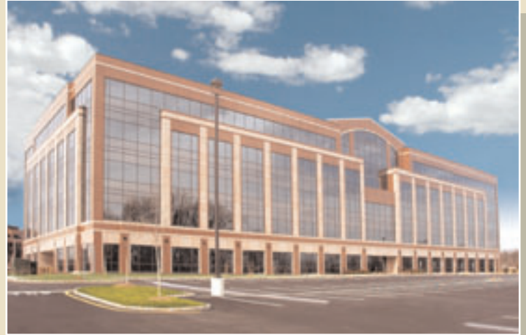
100 Kimball Drive Exterior
