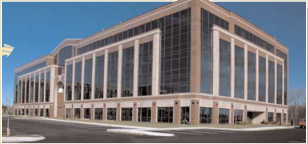
100 Kimball Drive Exterior
